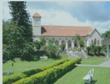
HOSPITAL SANTA TEREZA - SC
