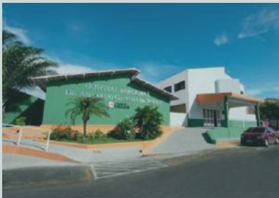
HOSPITAL MUNICIPAL DR. ABELARDO GADELHA DA ROCHA - CE
